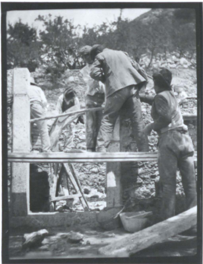
6.50 Erecting the jambs of one of the salone doors c.1906.
