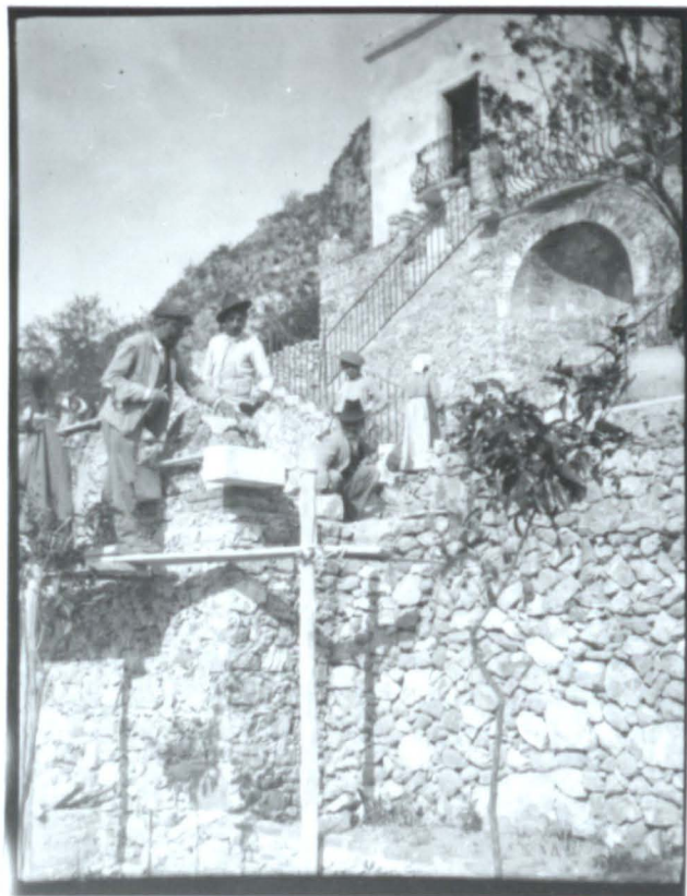
6.104 Constructing the machicolated tribune, Casa Cuseni , c.1907.
