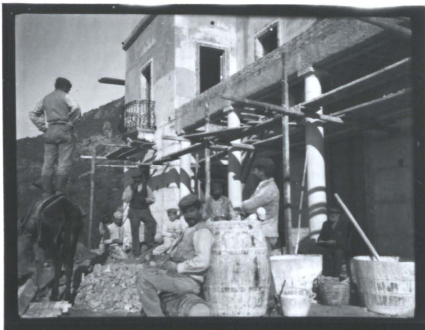
6.53 Slaking lime for the mortar and stucco of Casa Cuseni , c.1906.
