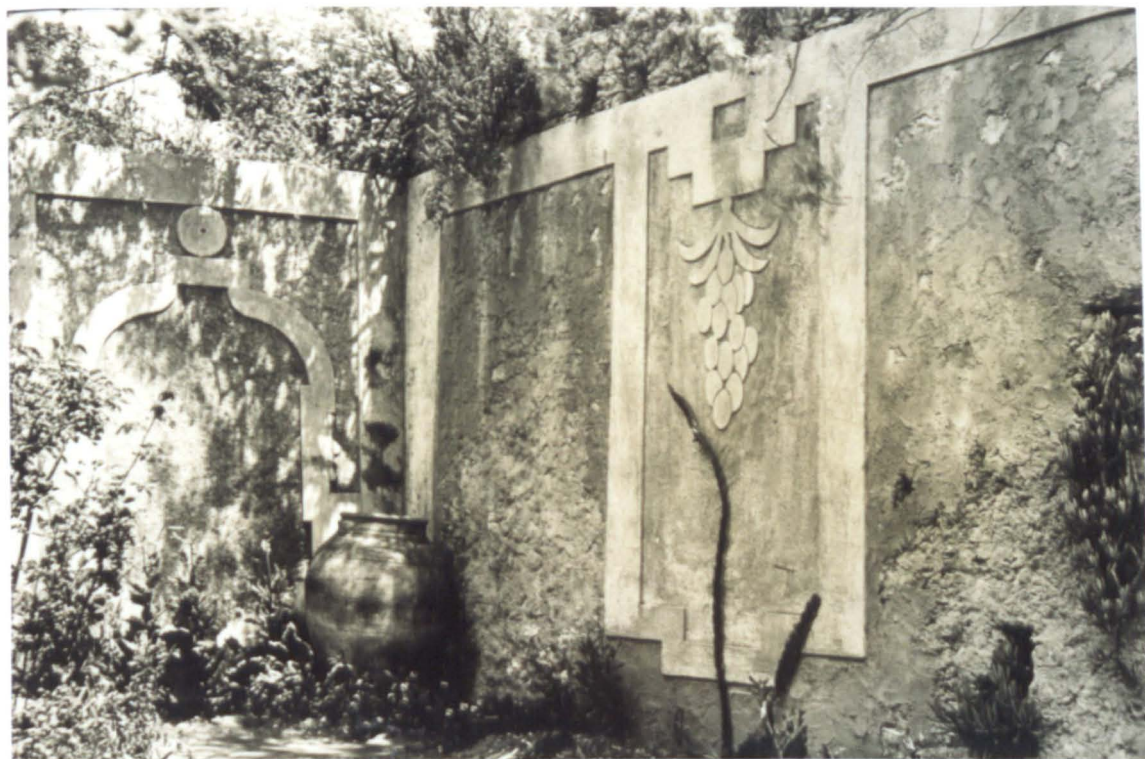
6.125 Stuccoed strapwork etc. on the retaining walls of the pozzo nero , Casa Cuseni, c.1932 but could be earlier.
