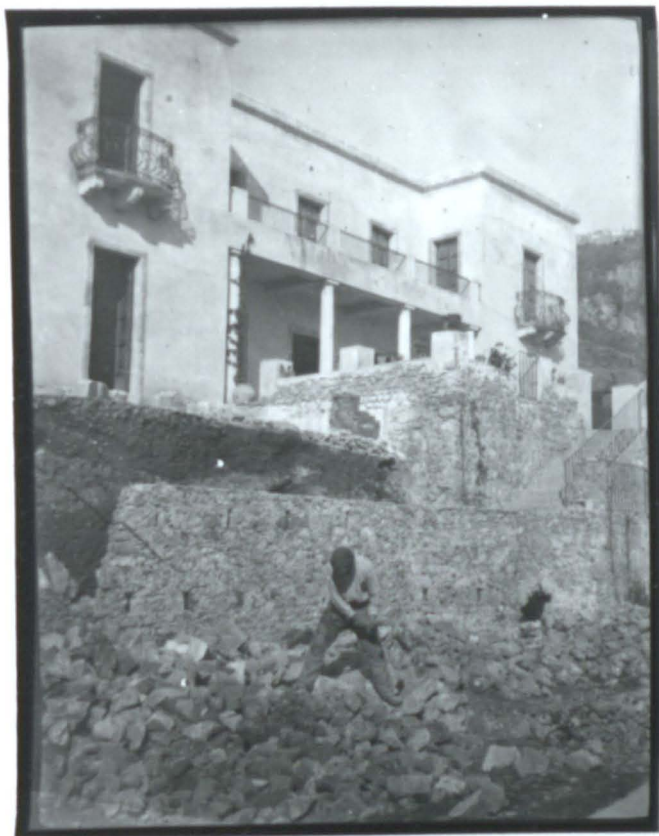
6.103 Building the retaining wall below the terrace of Casa Cuseni . c.1907.
