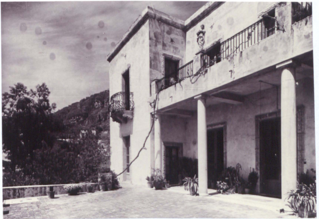
6.62 Front of Casa Cuseni , c.1932 The cistern underlies the terrace.
