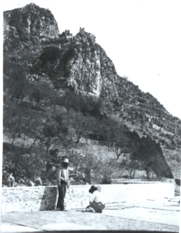
6.56 Sealing the roof of Casa Cuseni before tiling. Behind is the Rocca and Castello. c.1906.
