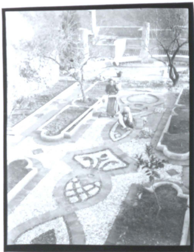
6.167 Laying the cobbles in the Ciottolato , Casa Cuseni.
