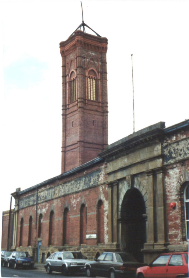
8.6 Tower Works, Globe Road, Leeds. Chimney based on Giotto's campanile for Florence Cathedral, 1899, by William Bakewell for Col. W.T. Harding, in 1994.
