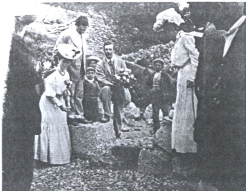
6.14 Ethel Kitson laying the foundation stone of Casa Cuseni in 1905, in the presence of the Siligatos and R.H.K. (Nino Siligato).
