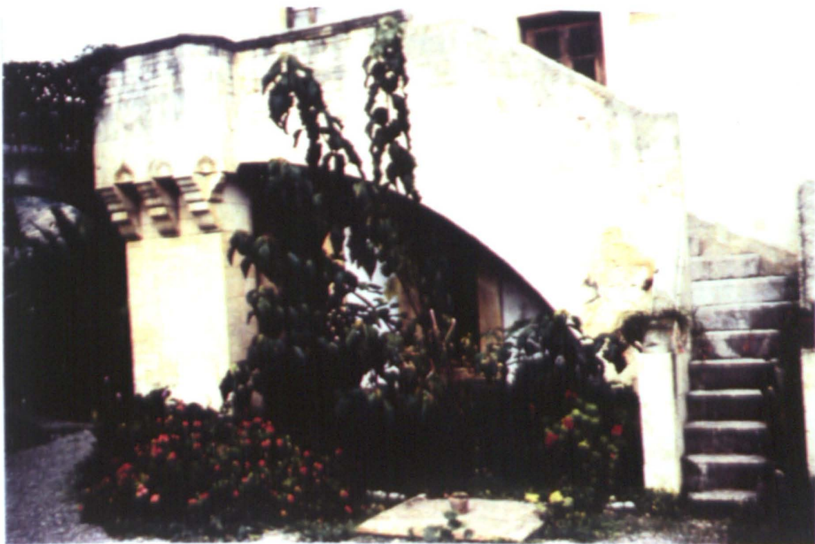
6.177 Staircase to minstrels' gallery and first floor, Villa San Giorgio, in 1981.
