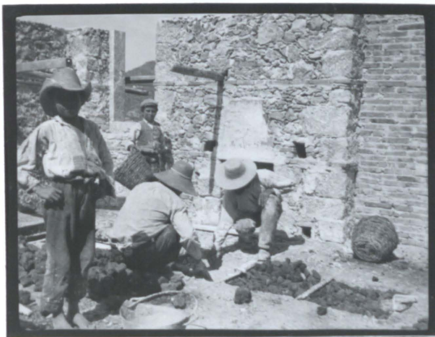
6.54 Insulating the first floor with larva between the r.s.j.s. c.1906.
