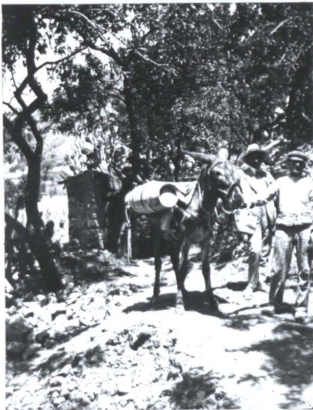
6.44 All the water for the building came from the Cuseni fountain below S. Francesco di Paolo.
